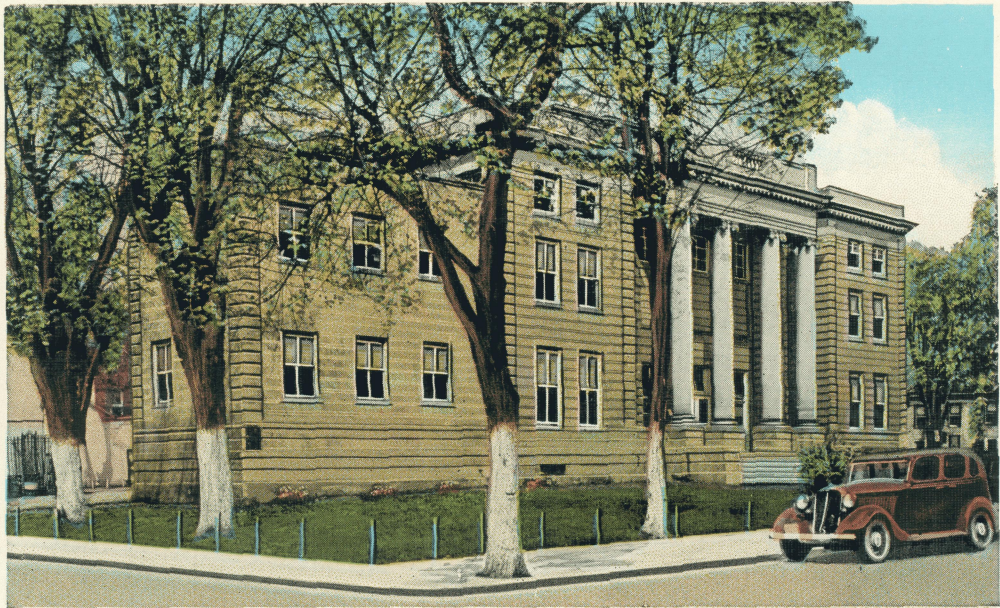
Municipal Building, Catlettsburg, Ky.
