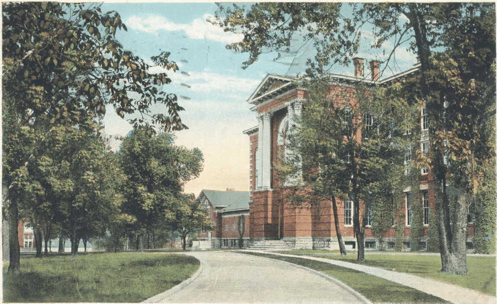
Main Building, Centre College, Danville, Ky.—2
