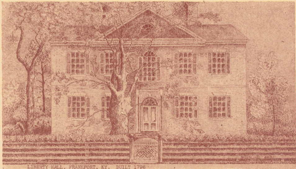
LIBERTY HALL, FRANKFORT, KY. BUILT 1796
