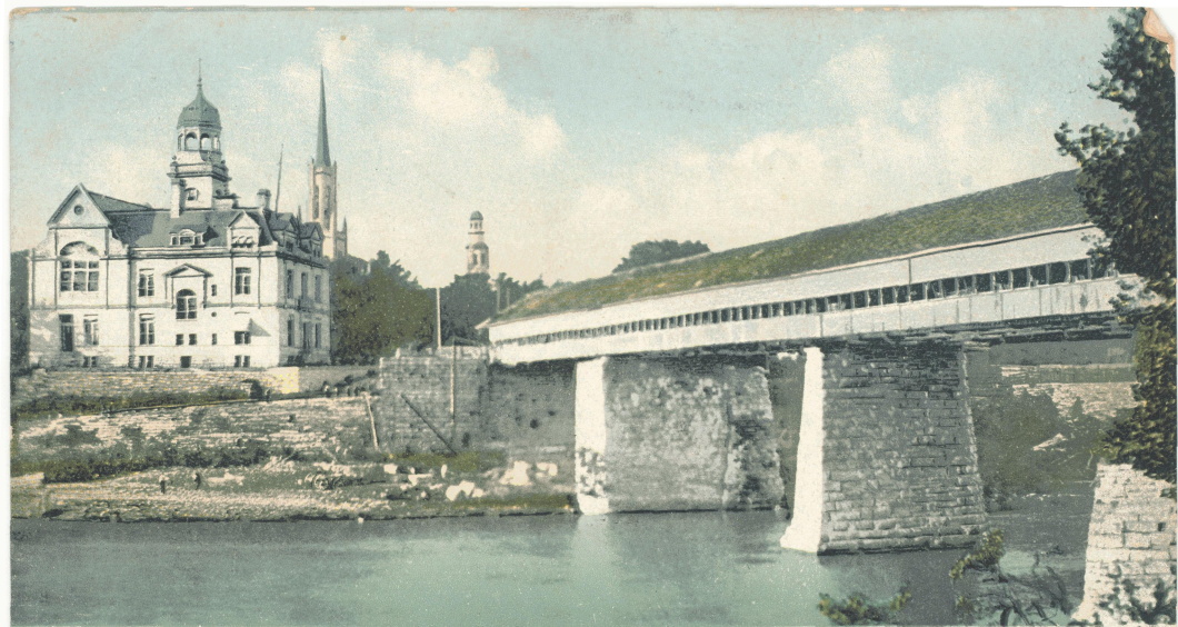
Custom House and "Old Wooden Bridge" over the Kentucky River
