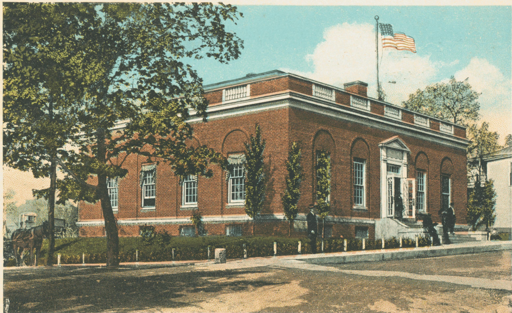
GOVERNMENT BUILDING AND POST OFFICE, GLASGOW, KY.
