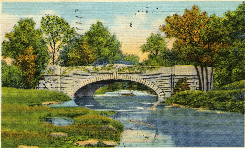
BELKNAP BRIDGE, CHEROKEE PARK, LOUISVILLE, KY.
