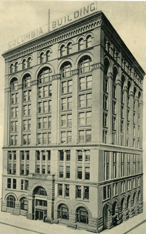
Columbia Building, Louisville, Ky.
