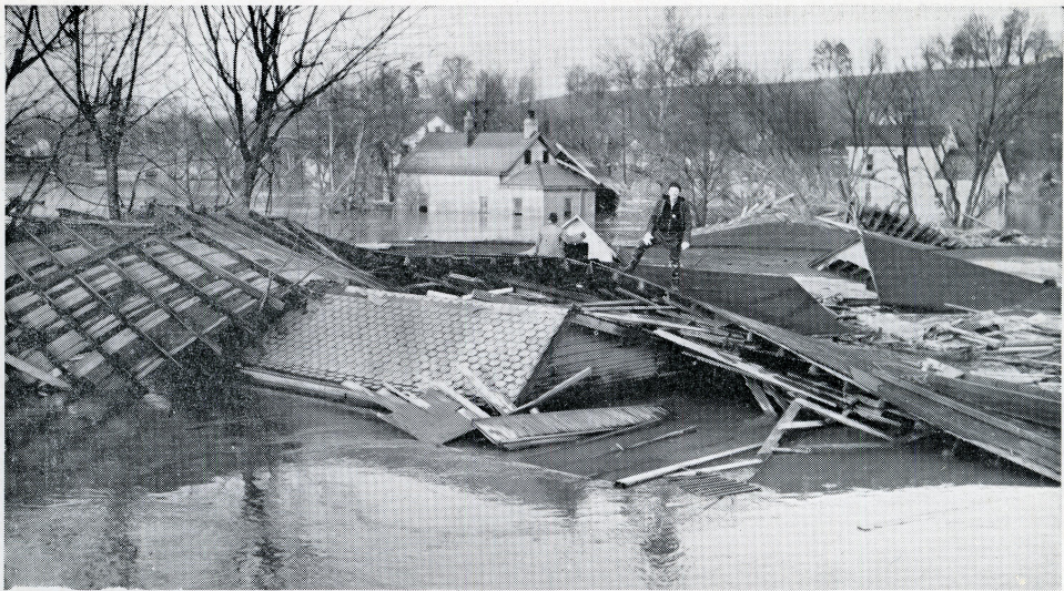
10763 Shippingport wreckage. This part of Louisville will be "parked" in future
