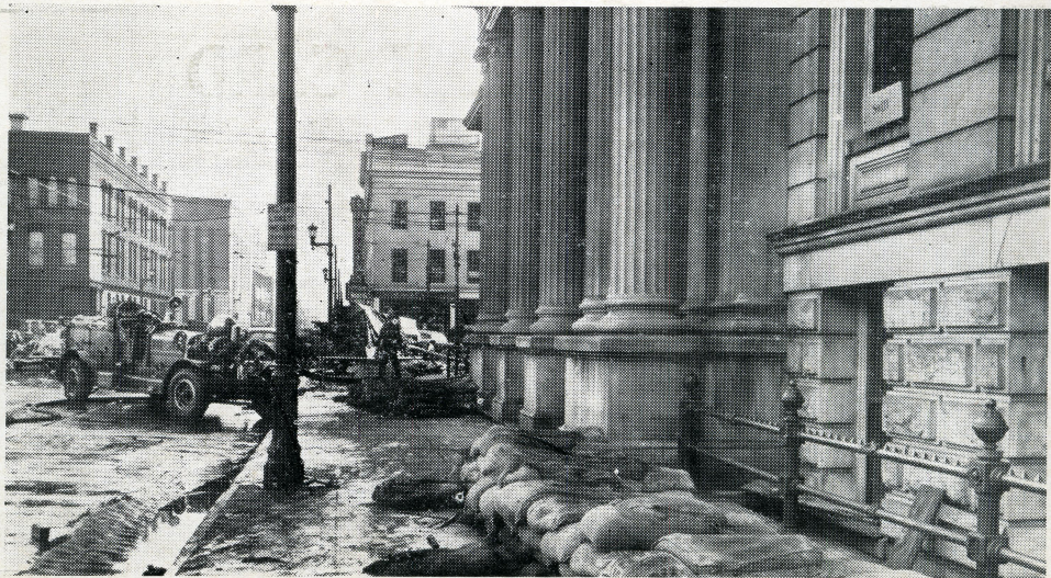
149475 City Hall sand-bagged to protect fire, police and telephone lines for rescue work
