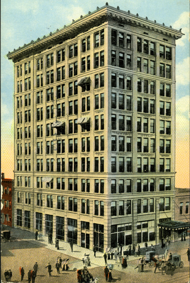
Realty Building, Louisville, Ky.
