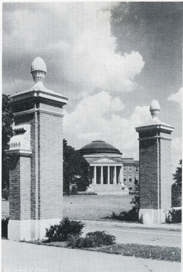
Administration Building, University of Louisville Belknap Campus, Louisville, Kentucky
