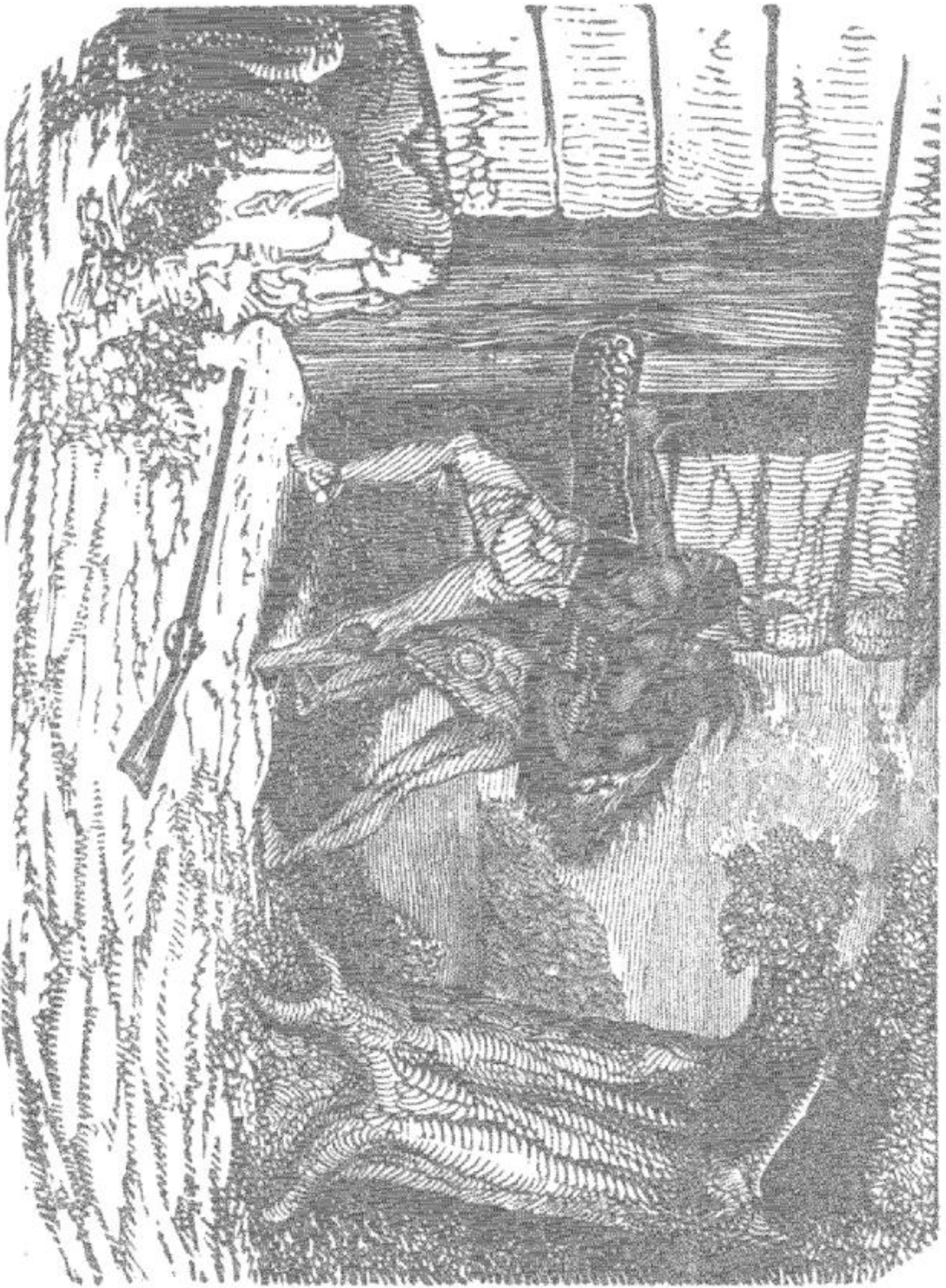
BREAKING INTO MR. STUART'S HOUSE.
