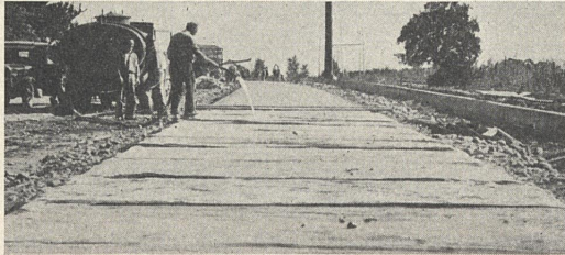
FIGURE 1.—COTTON MATS IN PLACE BEING WET DOWN.
