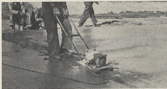
FIGURE 14.—CONCRETE FINISHING MACHINE, SHOWING PAN-TYPE VIBRATOR MOUNTED BETWEEN THE TWO SCREEDS.
