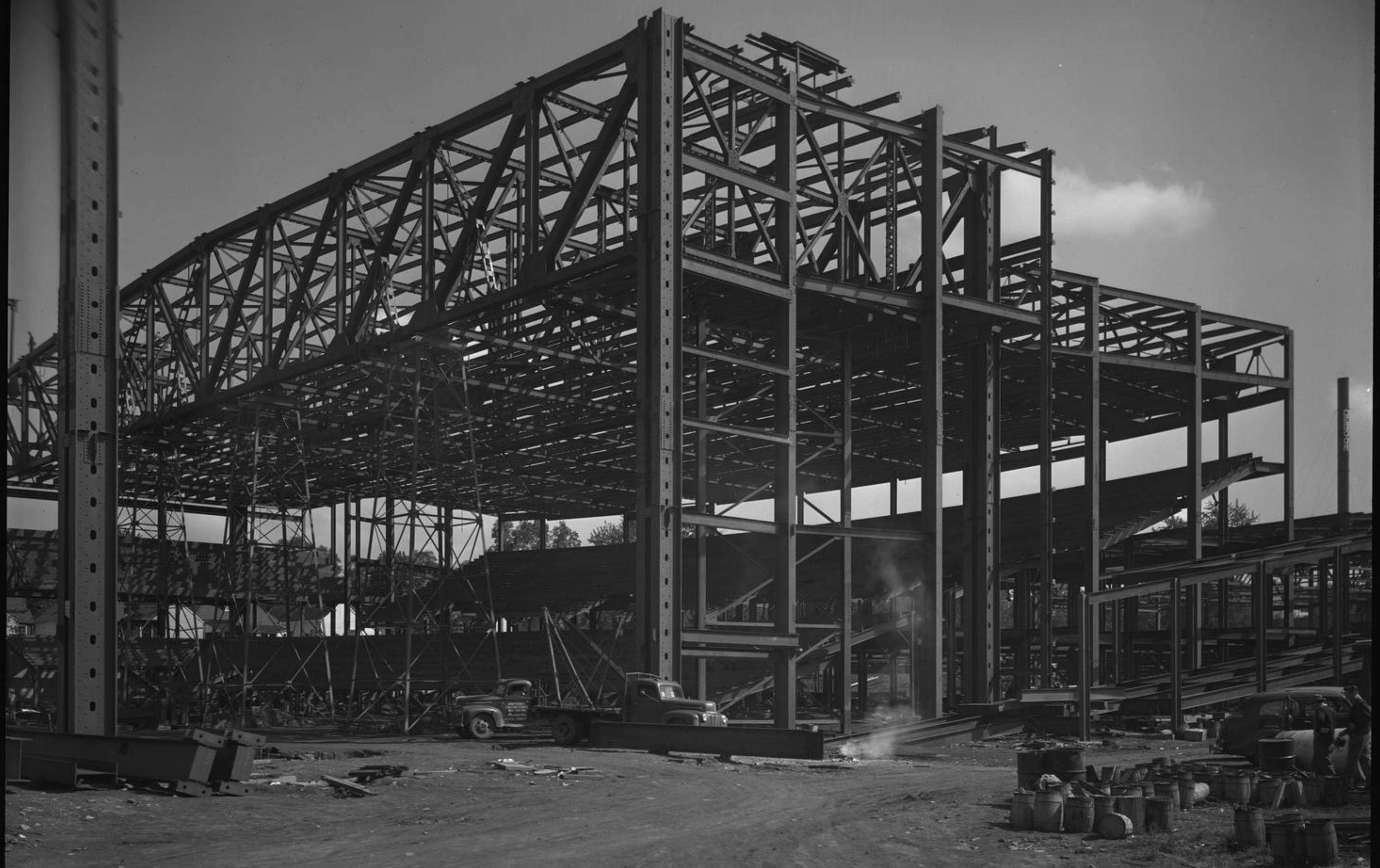
FIELD HOUSE -- LEXINGTON, KY MIDLAND STRUCTURAL STEEL CO. 10/5/48
