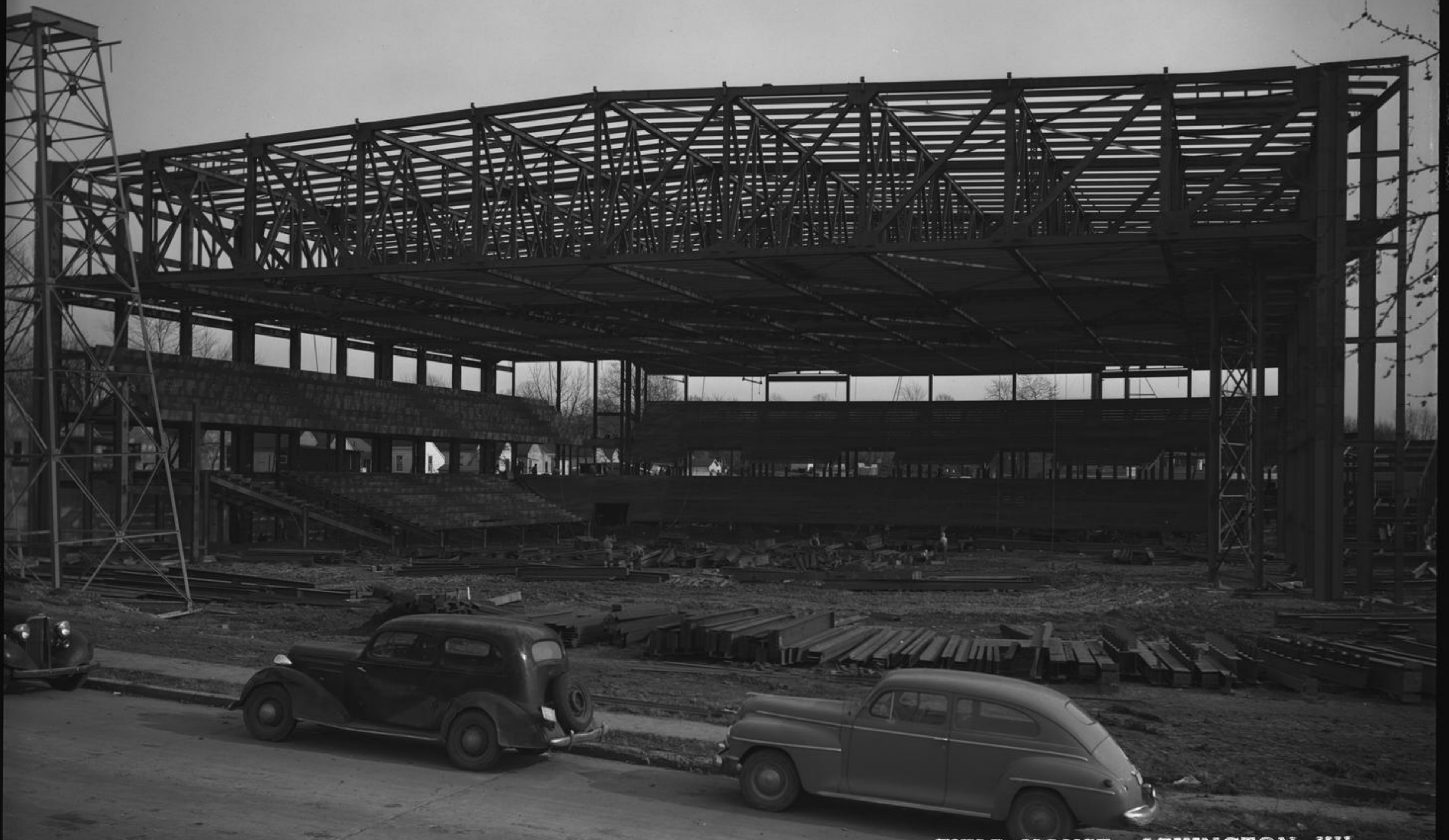
FIELD HOUSE -- LEXINGTON, KY. MIDLAND STRUCTURAL STEEL CO. 11/8/48
