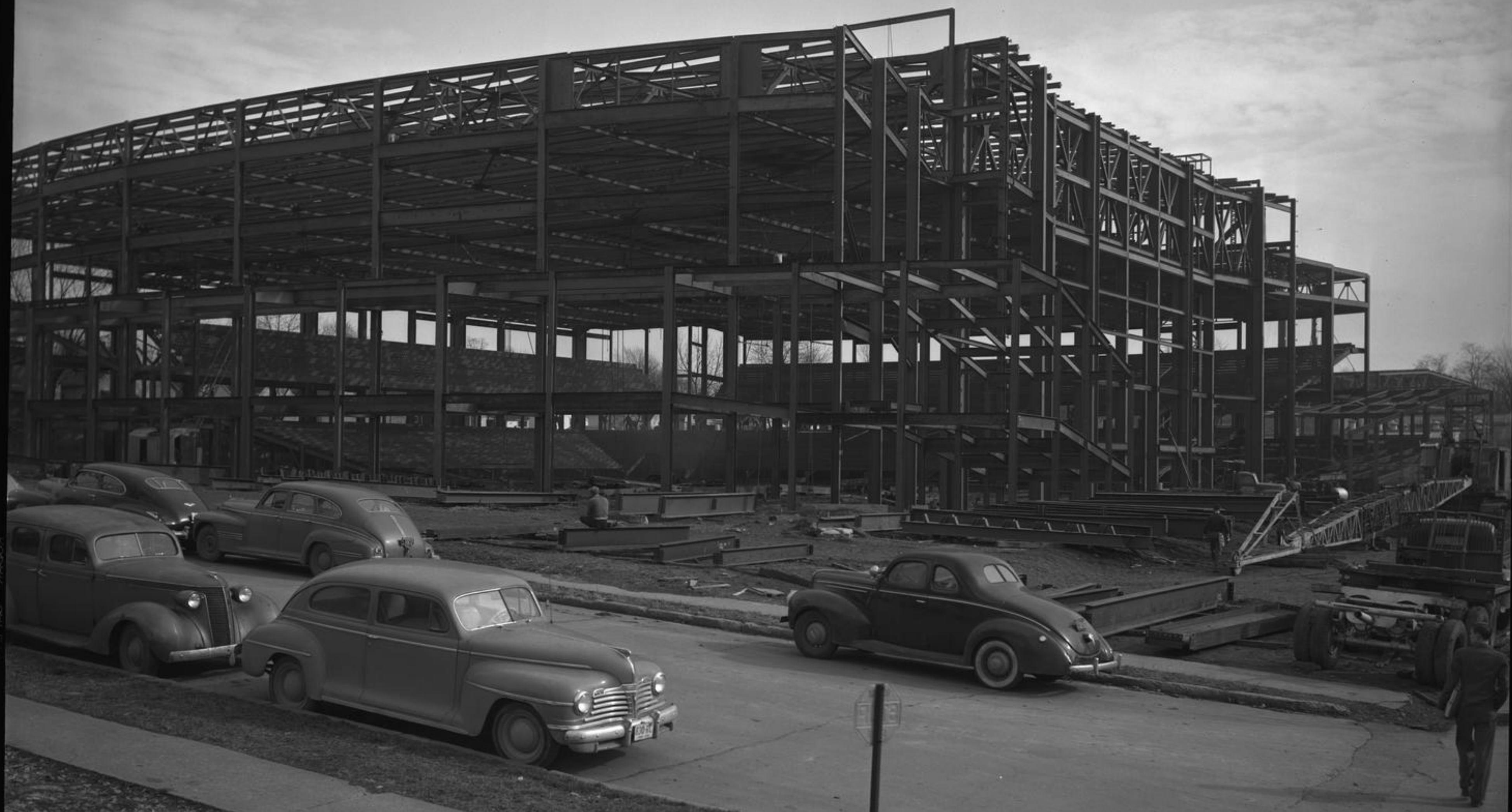
FIELD HOUSE -- LEXINGTON, KY. MIDLAND STRUCTURAL STEEL CO. 11/23/48
