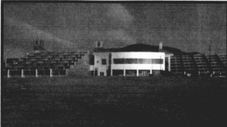
The National Renewable Energy Laboratory in Golden, Colo. The Solar Energy Research Facility is NREL's newest building on the South Table Mountain site. The SERF is designed to be the most energy-efficient building in the federal government and serves as a model for efficient office daylighting.
