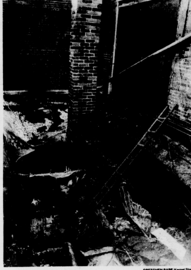
(left) The damage from Saturday's fire in Fleur-De-Lys restaurant caved in the roof. (right) Fred Mills, manager of the Kentucky Theatre, stands outside the box office. The theater will reopen in a couple of months.
