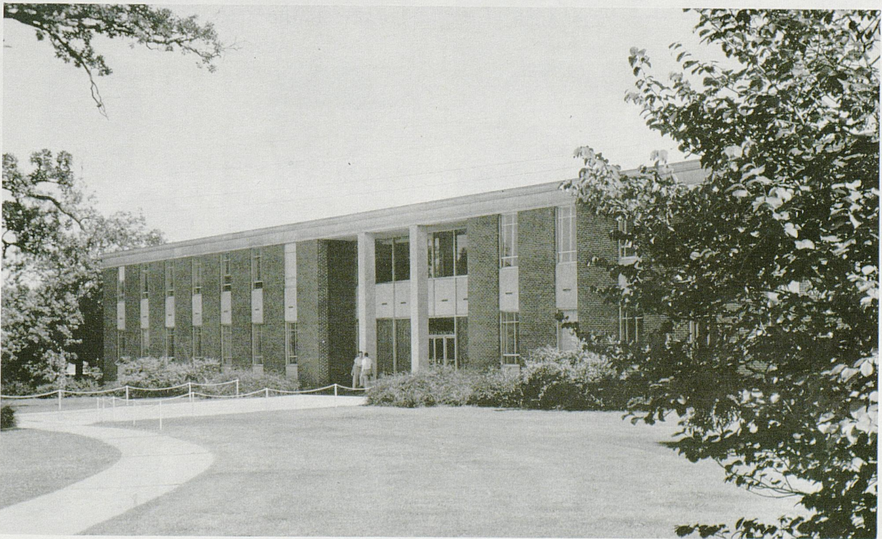
CARRIER ENGINEERING BUILDING
